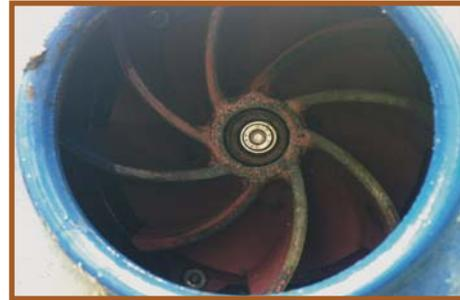
Rag-free pump impeller after 2 months of DERAGGER II operation
