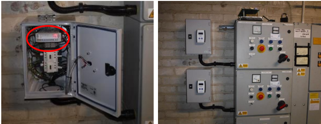
Photograph 3.2 Thorn Park installation of the DERAGGER
