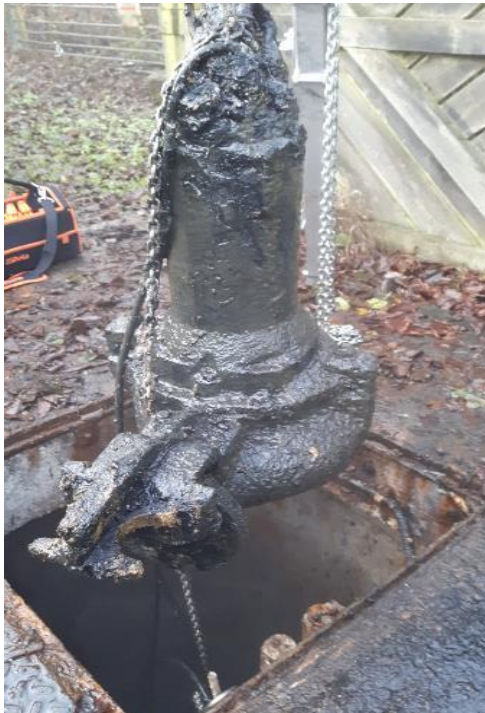
Photograph 4.3 Pump condition Navigation Way, pre-cleaning
