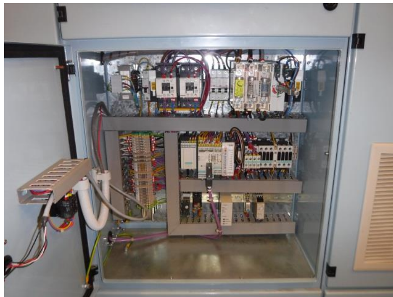
Photograph 3.1 Typical installation of the DERAGGER at Bridgewater West Quay, centre of middle rail
