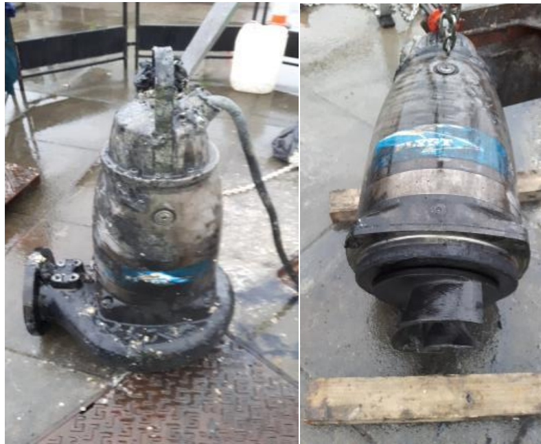
Photograph 4.2 Pump condition Dutton Forshaw, pre-cleaning
