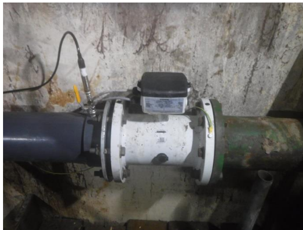
Photograph 4.1 Flow meter installation at Thorn Park
